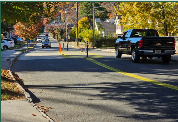
Figure 43. Plastic delineators marking the temporary median over the Peckman River Bridge, looking west.
