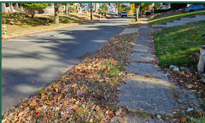
Figure 22. Uneven pavement.
