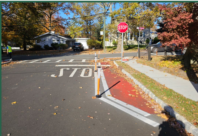
Figure 54. Plastic delineators marking the temporary curb extension on Derwent Avenue, looking north.
