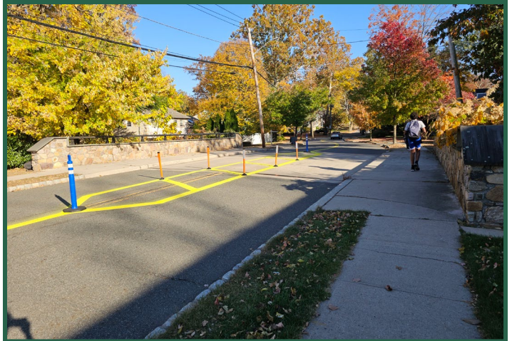
Figure 42. Plastic delineators marking the temporary median over the Peckman River Bridge, looking east.
