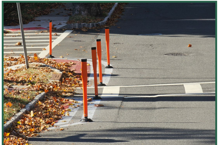
Figure 55. Plastic delineators marking the temporary curb extension on Linden Avenue, looking west.
