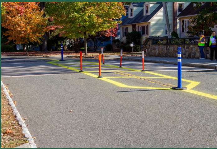
Figure 41. Plastic delineators marking the temporary median over the Peckman River Bridge.
