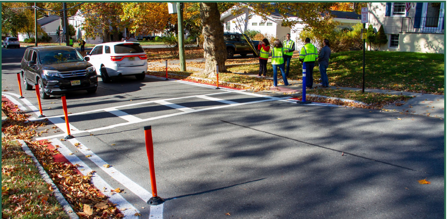
Figure 56. Two-way traffic passing the narrowed roadway with the temporary curb extensions.
