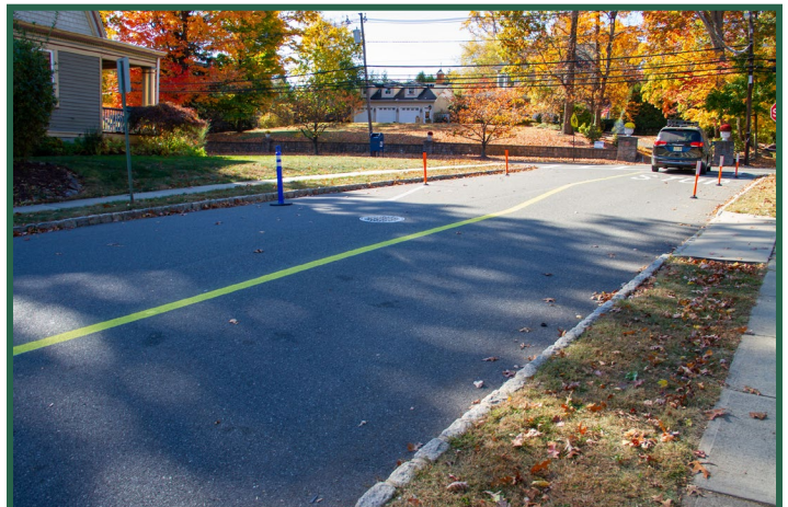
Figure 32. Plastic delineators located near the intersection with Fairview Avenue.
