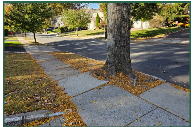
Figure 60. Uplifted sidewalk.
