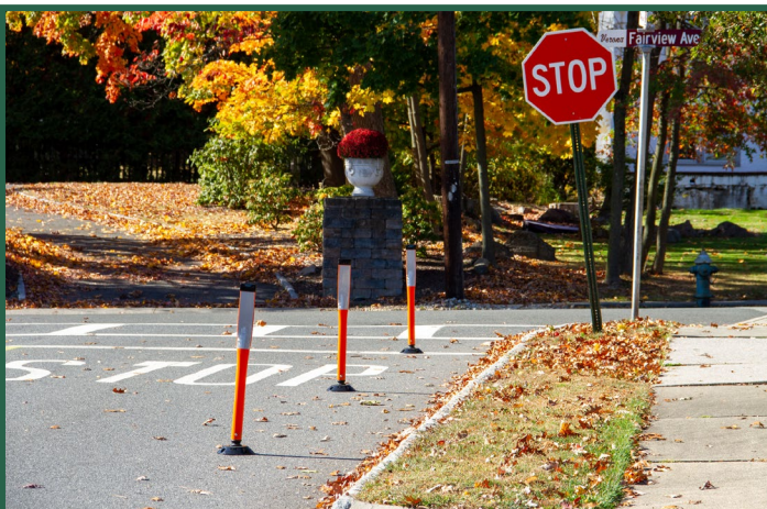
Figure 31. Plastic delineators located near the intersection with Fairview Avenue.
